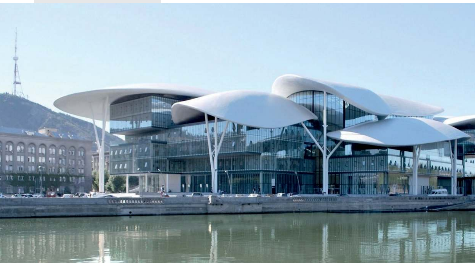
Tbilisi Public Service Hall Tbilisi, Georgia Studio Fuksas
